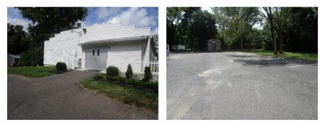
The section of parking spaces on the south side of the property can be replaced with pervious pavement to capture and infiltrate stormwater runoff from the parking lot. A preliminary soil assessment suggests that the soils have suitable drainage characteristics for green infrastructure.
